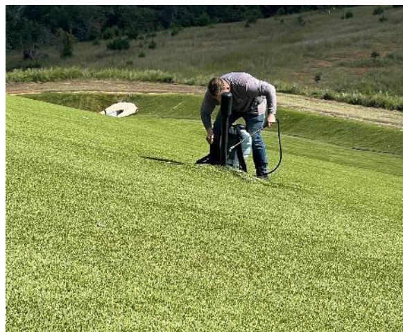
Figure 6. DuraGuard® and infill application after bird damage repair at PRV
