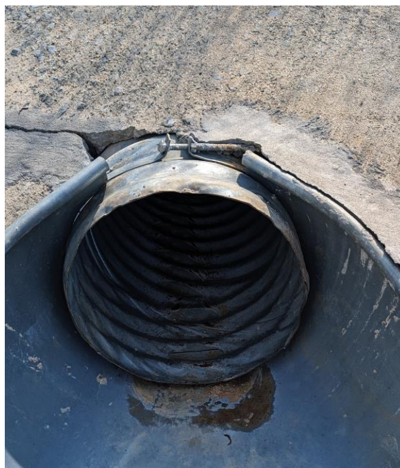
Photo 6 – Storm Water Inlet Structure
