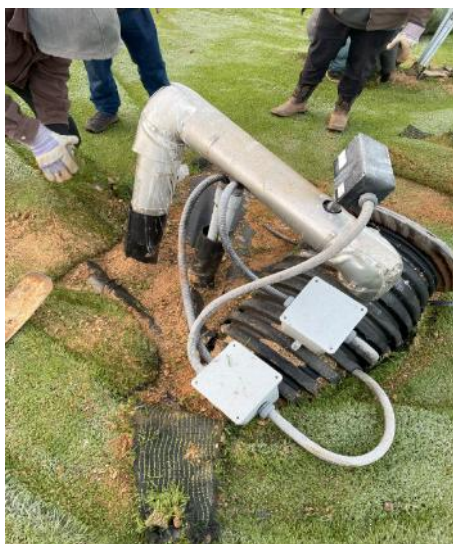
Figure 9. Settlement induced wrinkles and torn Closuresurf® at leachate piping on south slope
