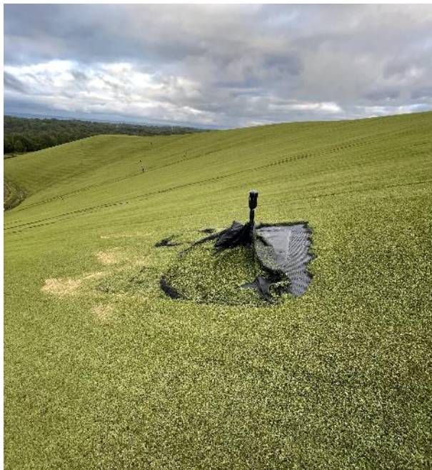
Figure 1. Bird damage around PRV
