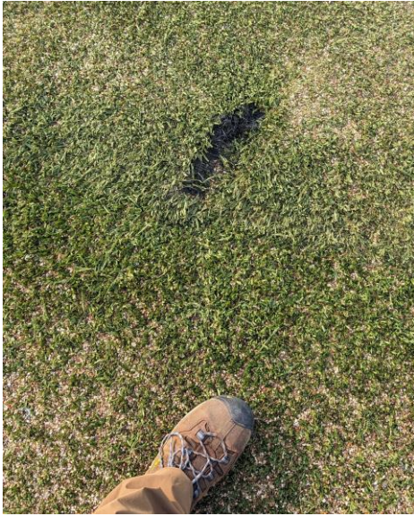
Photo 1 – Bird Damage of Engineered Turf
