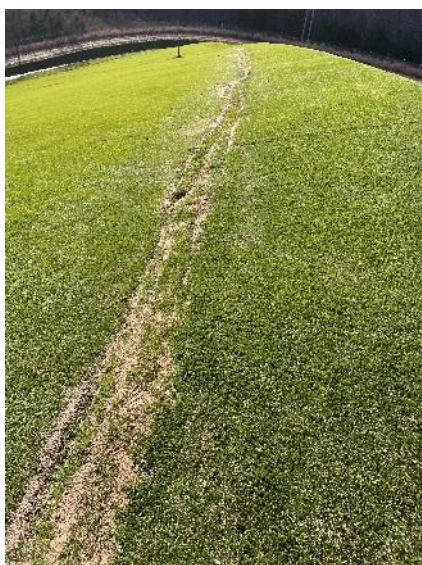
Figure 11. Seam repair on Cell 1-2
