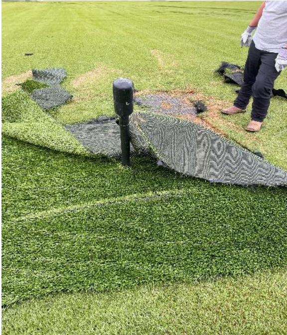
Figure 3. Repairing bird damage around PRV
