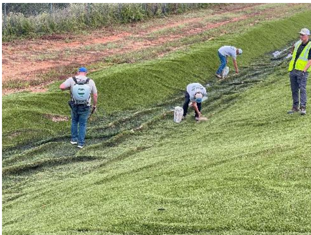
Figure 5. DuraGuard® and infill application to wrinkles
