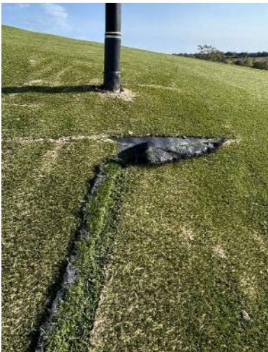
Figure 7. Bird damage at gas well
