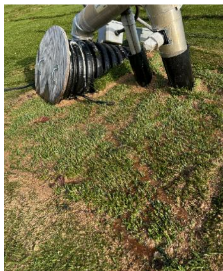
Figure 10. Repaired wrinkles and torn Closuresurf® at leachate piping on south slope
